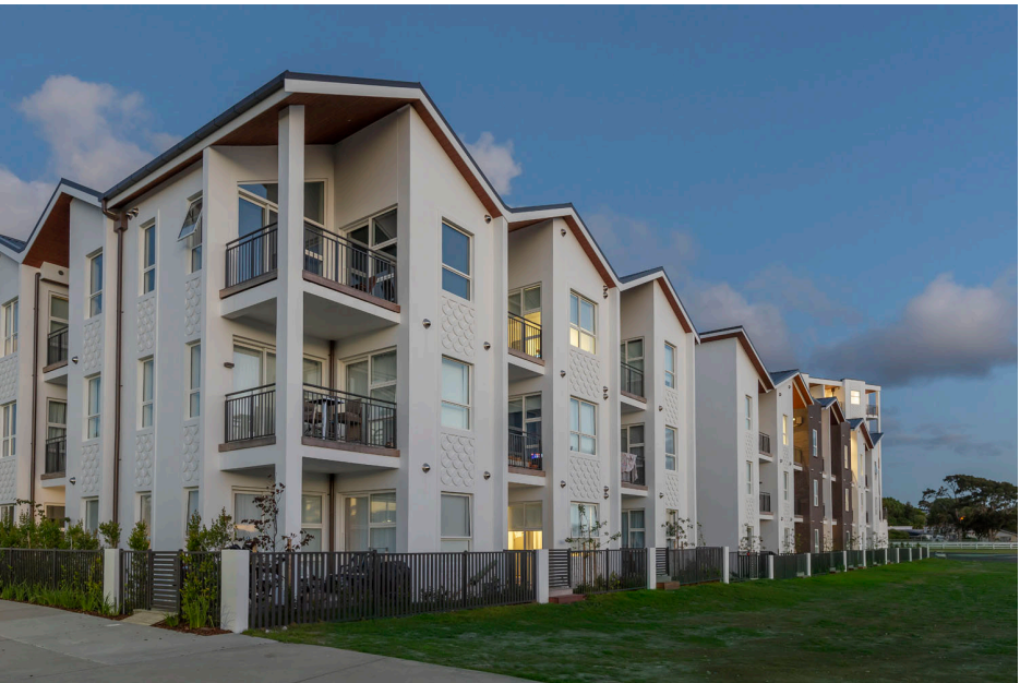
Walk-up apartments using gabled-roof form and modulation to read as terraced housing (Example 2)
