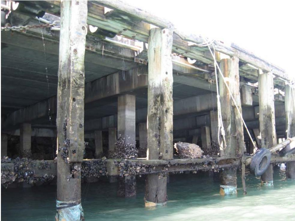
**Photograph 11:** Showing large section loss in horizontal timber member of fender system.
