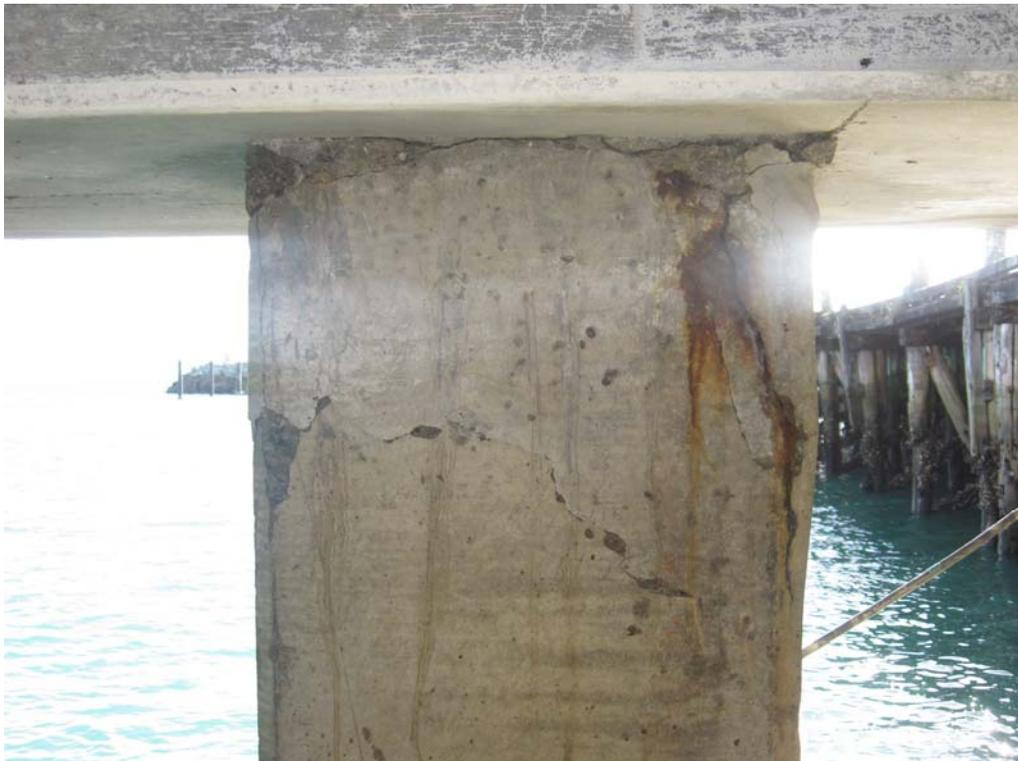
**Photograph 6:** Typical spalling of concrete at top of piles.
