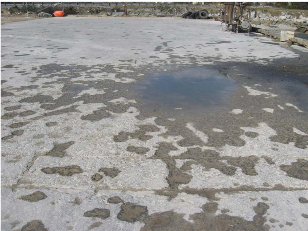
**Photograph 2:** Abrasion to surface of wharf. Probably caused by placing and moving large rock or mussel farm anchor blocks across the wharf.
