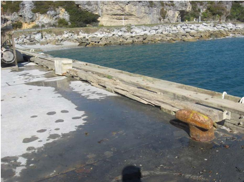
**Photograph 4:** Damaged timber kerbs.
