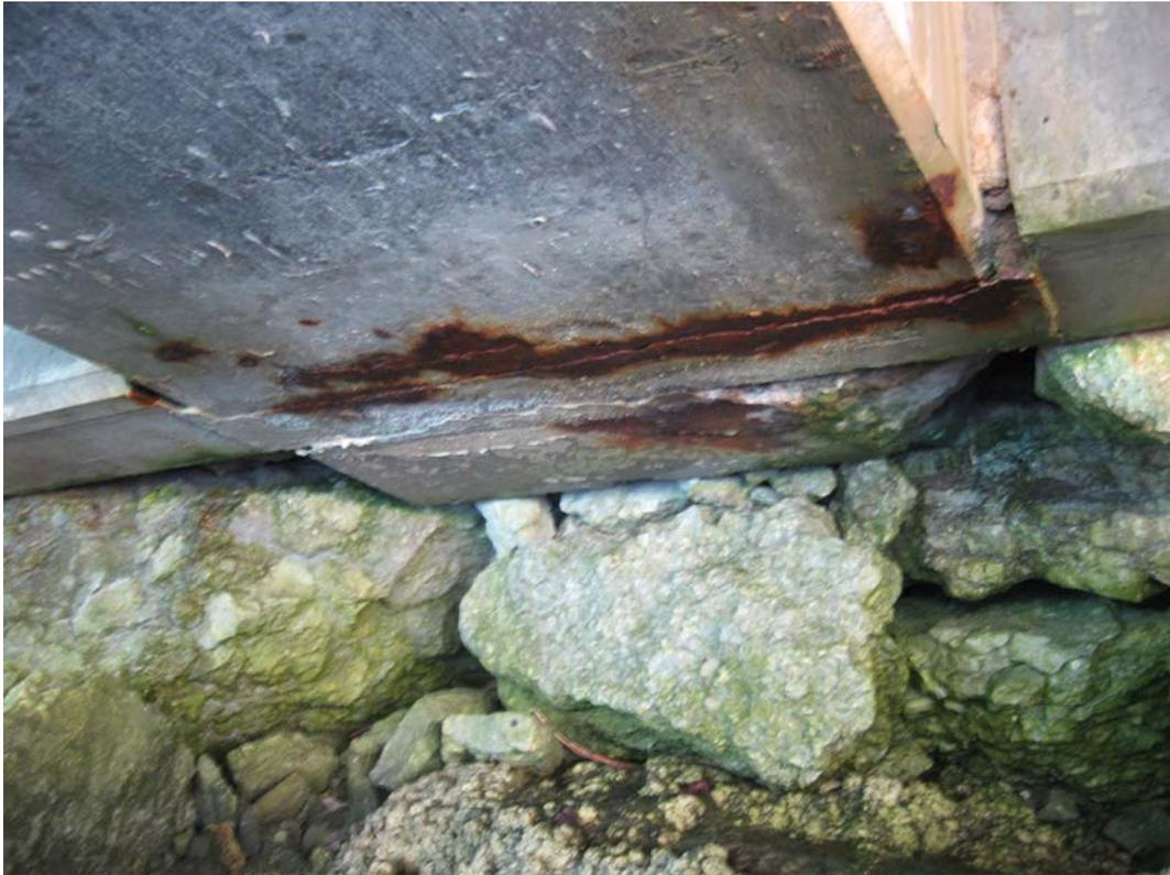
**Photograph 9:** Typical cracking and rust staining to underside of beam joint on landward side of wharf.
