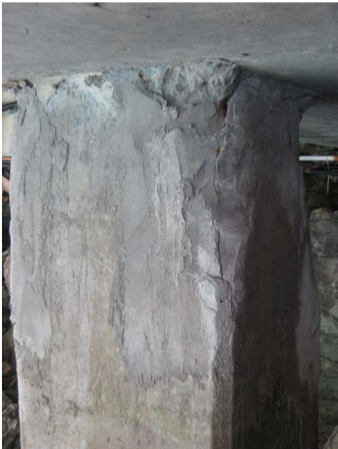
**Photograph 8:** Previous repair to top of concrete pile which has continued to crack and rust staining is visible.
