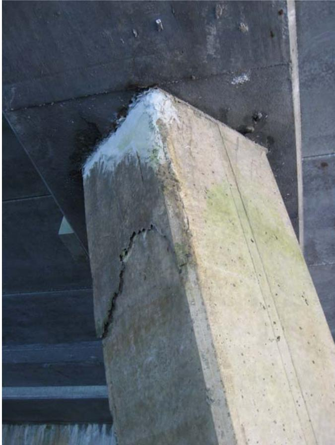
**Photograph 7:** Typical spalling of concrete at top of piles.
