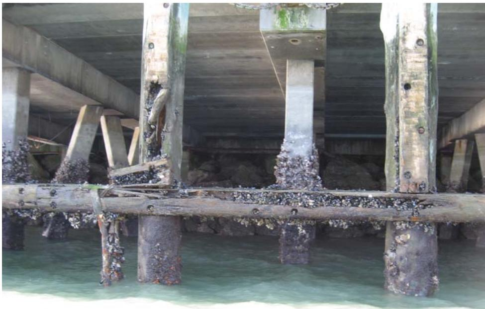
**Photograph 12:** Badly decayed horizontal timber post in fender system. Also bad decay in left hand fender system timber pile.
