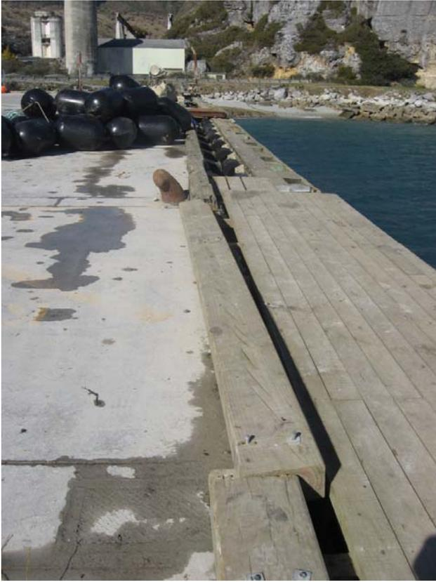
**Photograph 3:** Loose timber kerb at edge of wharf.
